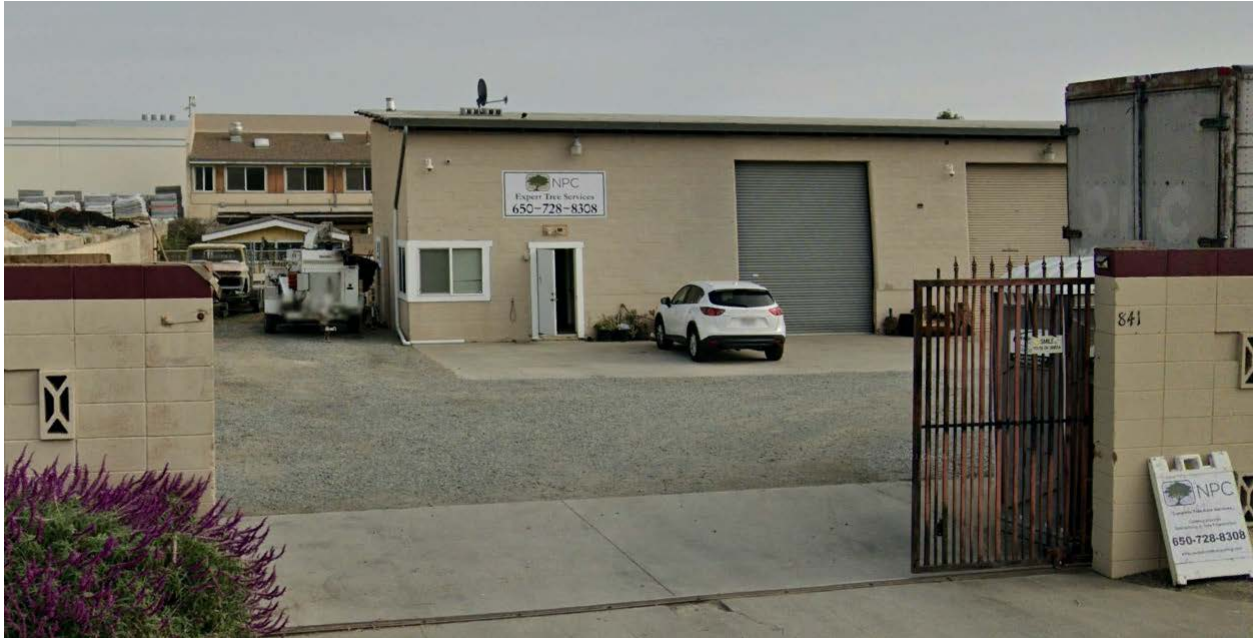
Fig.12 – 841 Old County Rd. – Front (west), from Old County Rd.
